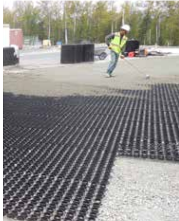
Grass Paver Fire Lane Installation
