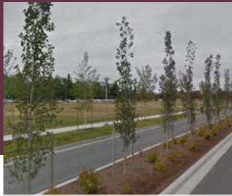
Example of median with green infrastructure
