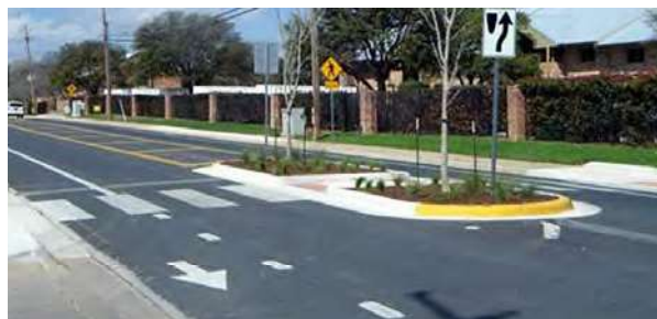
Figure 9. Midblock crossing island as part of a continuous median (left) or as a stand-alone feature for an intersection (right) (image source: Toole Design Group).
