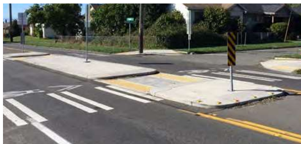
Figure 9. Midblock crossing island as part of a continuous median (left) or as a stand-alone feature for an intersection (right) (image source: Toole Design Group).
