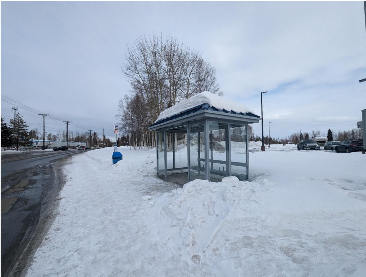
Figure 34 - MACS Bus Shelter
