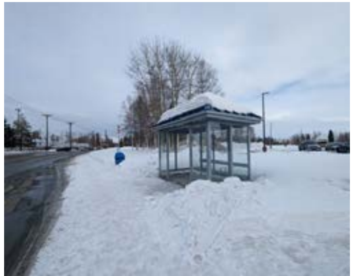
Figure 19: MACS Bus Shelter
