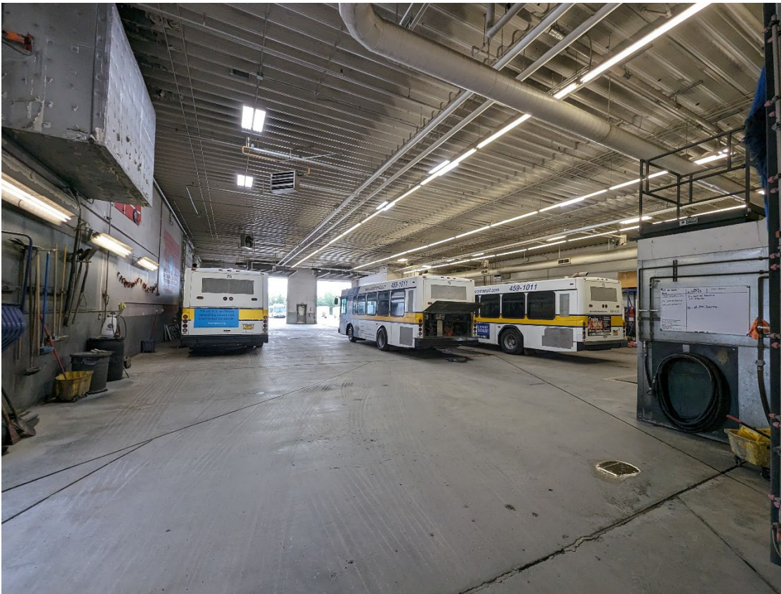
Figure 18 – MACS bus undergoing maintenance at agency facility
